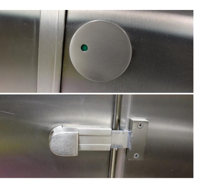
Locking and unlocking door automatically changes color of lock indicator
