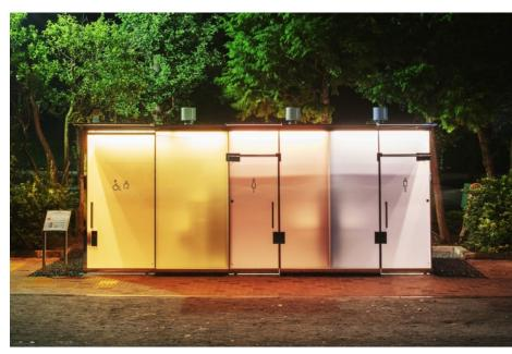
"There are two things we worry about when entering a public restroom, especially those located at a park. The first is cleanliness, and the second is whether anyone is inside. Using the latest technology, the exterior glass turns opaque when locked. This allows users to check the cleanliness and whether anyone is using the toilet from the outside. At night, the facility lights up the park like a beautiful lantern." – Shigeru Ban, Architect
